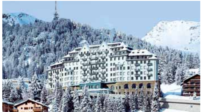
In the 5 star Ritz Carlton Hotel in St Moritz, heat is recovered from waste water.
